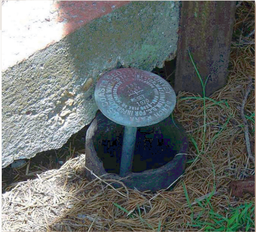
http://celebrating200years.noaa.gov/foundations/leveling/image8.html This elevation benchmark shows the effect of subsidence.
